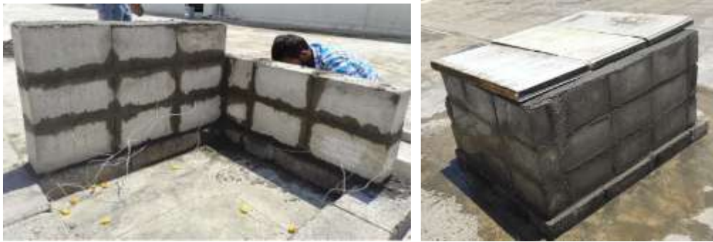
Trombe Wall Construction
